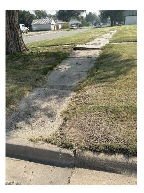
Photo 1: Example poor sidewalk condition, non-ADA compliant
